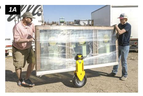
Make sure the load stays upright, with a minimum angle of tilt (fig. 1B).
