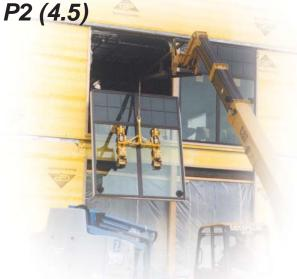
Employing a unique system of interchangeable lift frames and pad channels, these Powr-Grip® vacuum lifters conserve resources while supplying maximum versatility in a variety of work settings.
